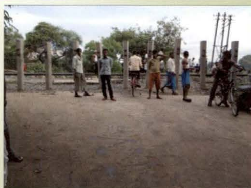
Connectivity was not provided to habitation because road was blocked by cement concrete pillars on both sides of railway track (in package no - BR-06R-148, Bhagalpur district, Bihar)
