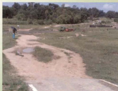
Habitation Kumhardab (Jashpur district, Chhattisgarh), was not provided connectivity due to non-construction of long span bridge
