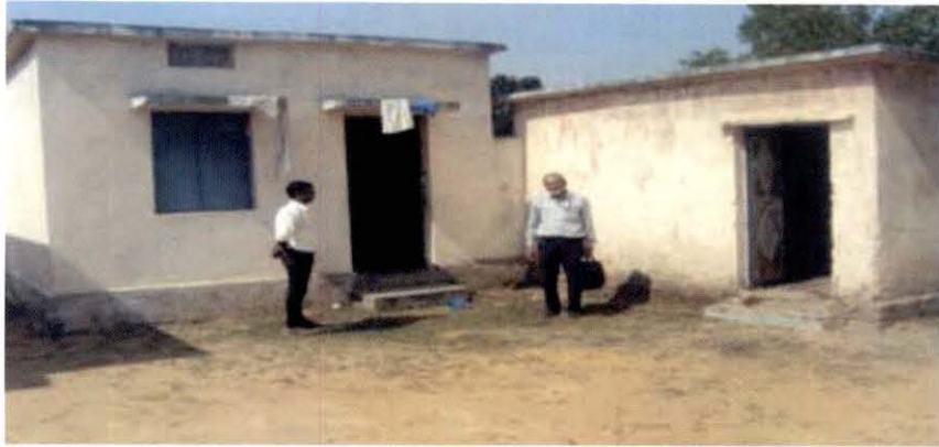
Photo 11: Multiple kitchen sheds constructed at Primary School Moliyatola, Anuppur, Madhya Pradesh dated 01 November 2014
