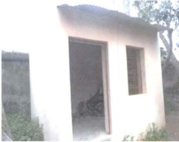
Photo 17: Cooking of MDM was not done in the newly constructed kitchen shed due to small size(10'X9')
