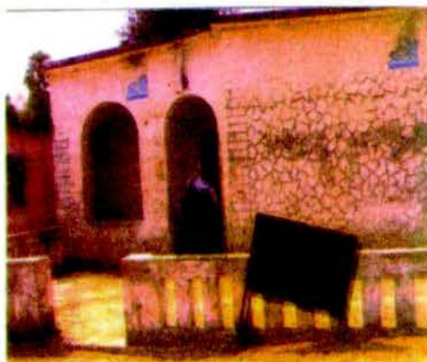
Closed Anganwadi Centre at Bangra Panchayat, Samastipur Date: 13-04-2007 at 10.09 AM
