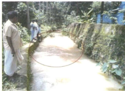
Photograph in Vattamankavu Temple taken on joint site visit, which shows no such structure
