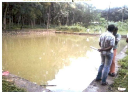
Renovation of ponds
