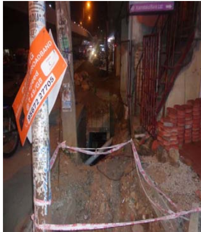
C-05&06 - CH: 2+070 to 2+170, (RHS) (25/07/2017)
