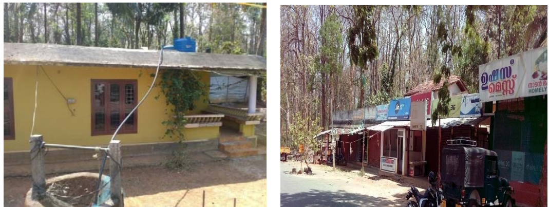
Pic 1&2 – Buildings illegally constructed in the erstwhile leased land near Muthanga checkpost in the Wayanad Wildlife Sanctuary. (Both pictures taken on 09 March 2018)
