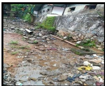
Pic.3: Waste water overflowing Kumbalamthodu
