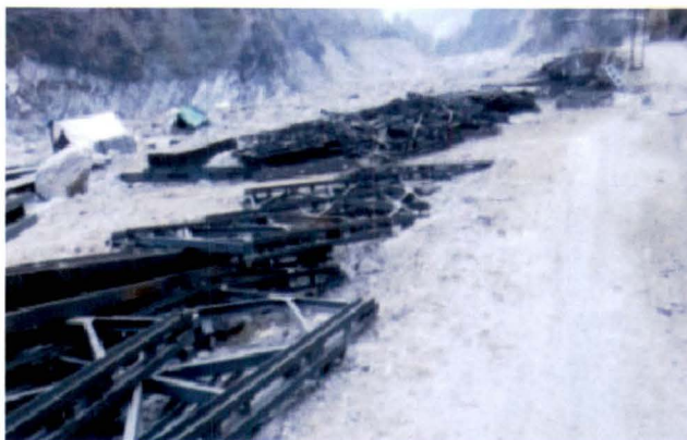
Material lying idle at construction site of Kanchoti (Pithoragarh) of 03.01.2015
