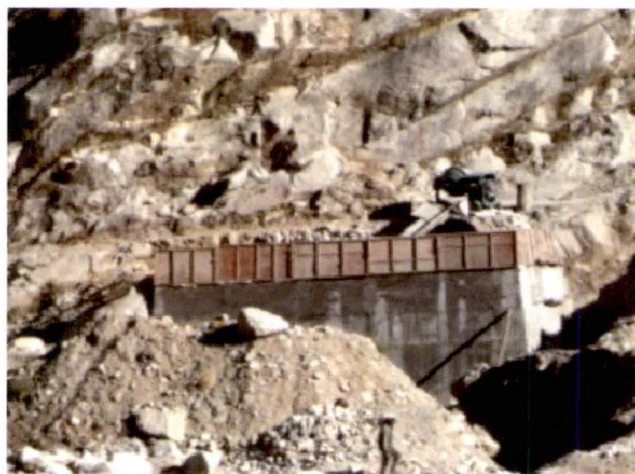
Fresh steel deck suspension bailey bridge at Kanchoti (Pithoragarh) of 03.01.2015
