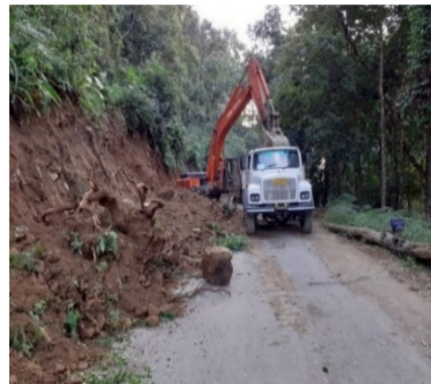
State Highway from Manpur to Nayabazar
