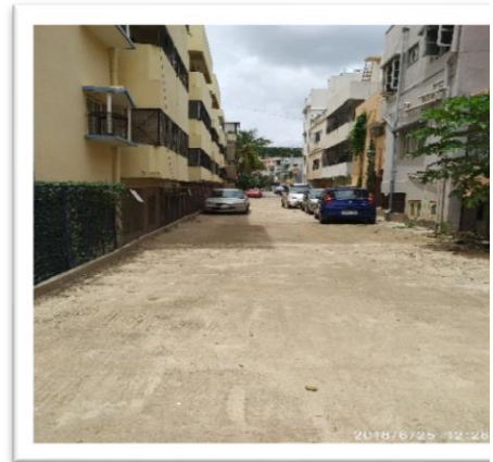
South Zone (Covered Drain)
