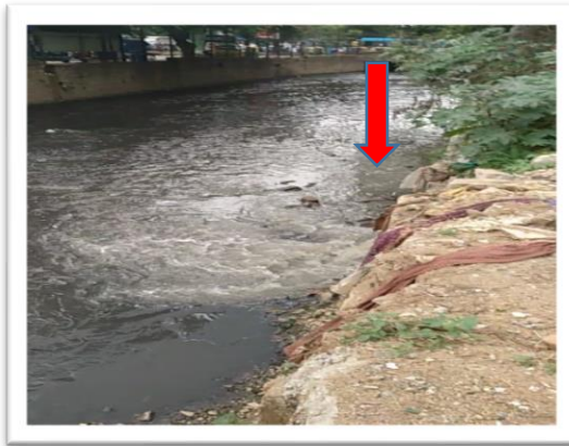
Discharge of sewage into SWD through BWSSB pipeline at Silk Board Junction, Bommanahalli Zone
