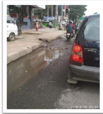
Exhibit 4.8: Photographs showing unscientific construction of roads/drains – absence of proper gradient/alignment
