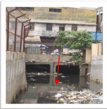
Private property on JC Road, Koramangala Zone
