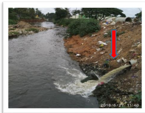
Direct discharge of sewage into SWD at Pattanagere, RR Nagar Zone
