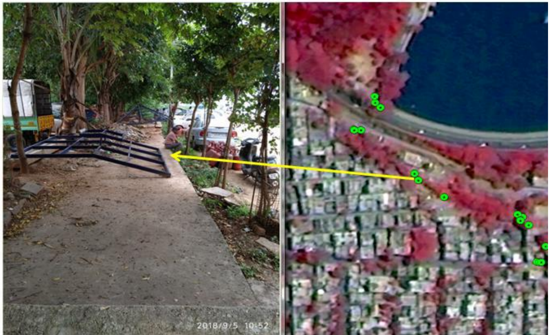
Covered drain adjacent to Sankey tank
