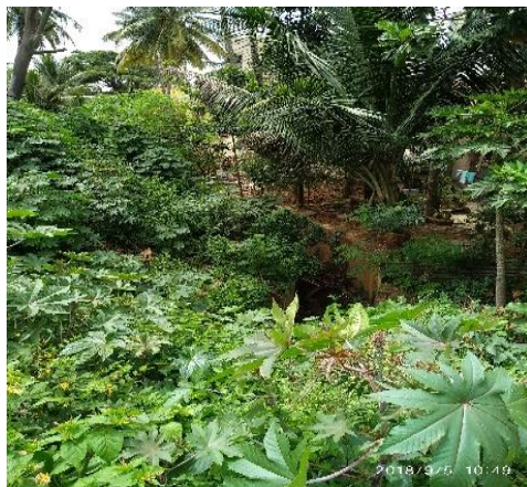
Vegetation inside SWD at Vyalikaval, West Zone
