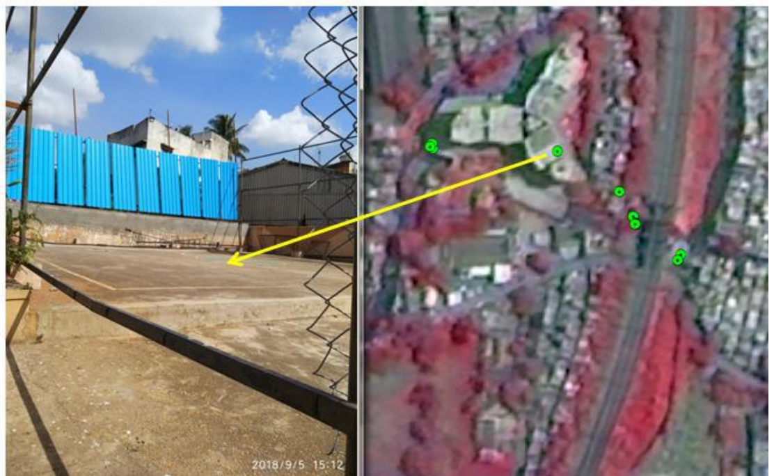
Drain encroached and covered by an apartment
