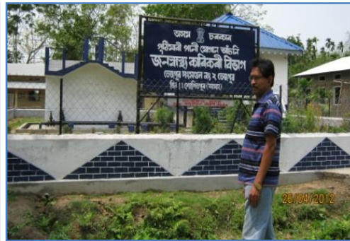
Completed scheme of Puthimari PWSS (26-04-2012)
