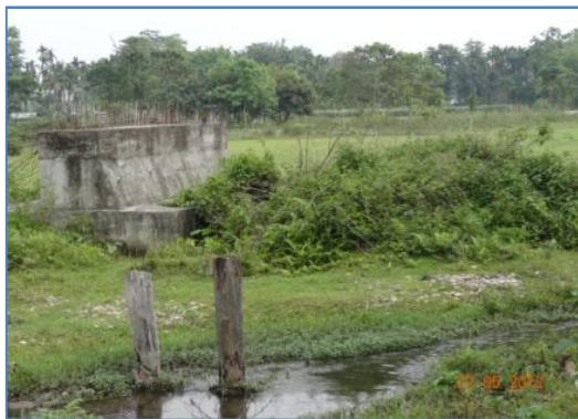
Incomplete RCC Bridge No. 5/1- Package No. AS-22-27 (27-05-2012)
