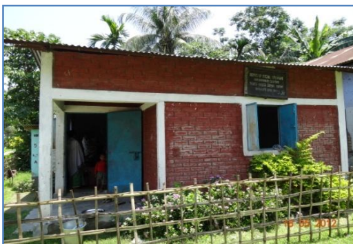
Anganwadi Centre No. 118 at Balikuthi running without water supply (15/05/2012)
