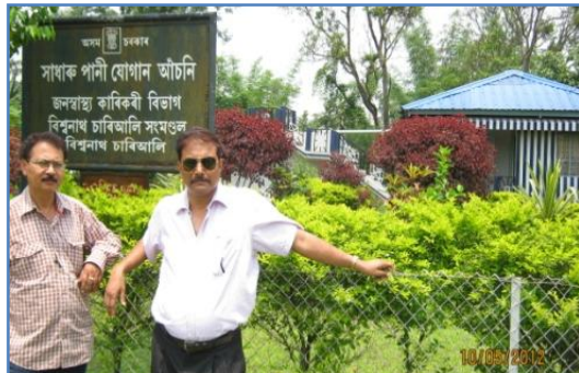
Completed scheme of Sadharu PWSS (10-05-2012)
