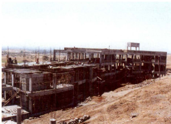
Incomplete administrative building
