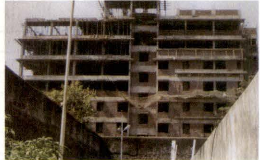
Highrise residential building under construction near Mumbai Central Prison
