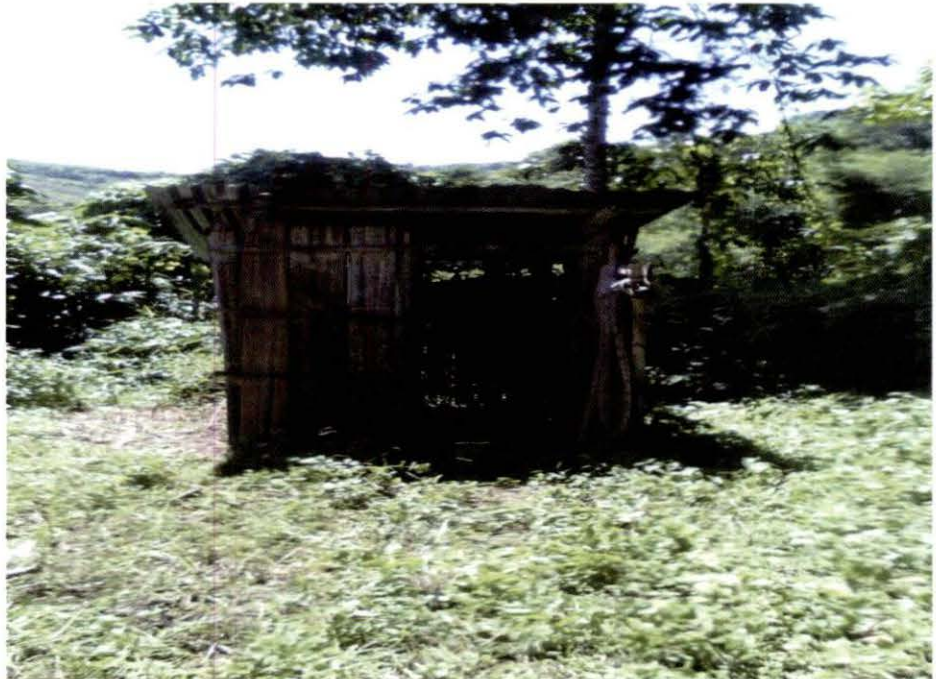
Anganwadi Toilet at Khamlang GP Nampong Block, Changlang district, Arunachal Pradesh
