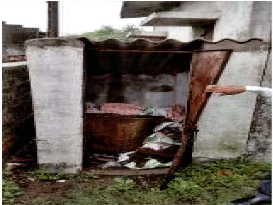
Anganwadi Toilet in Adol GP, Ankleshwar Taluka, Bharuch district, Gujarat
