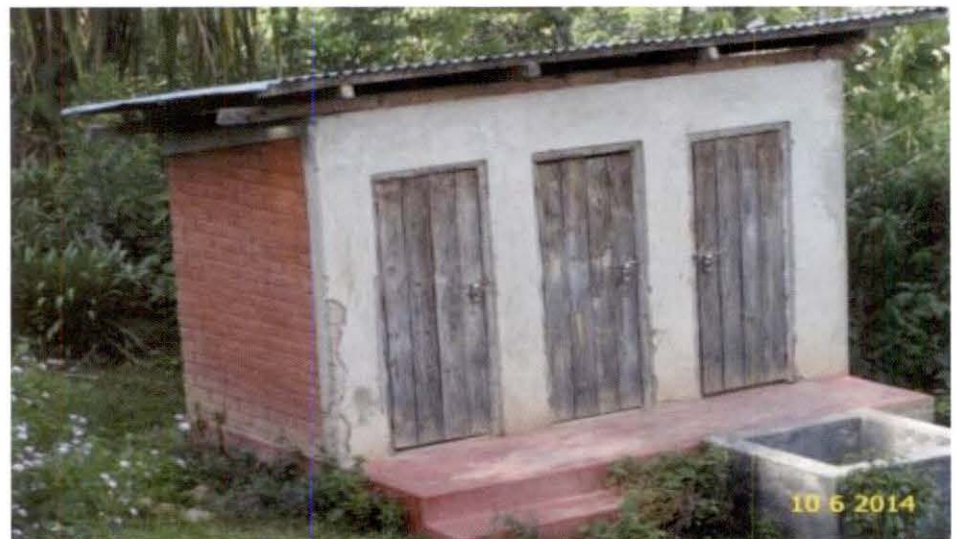
CSC without prescribed facilities at Sandangshenba Maring village under DWSM Kangpokpi Manipur !
