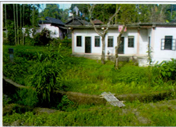
Photograph – 2.2.4 Unutilised community halls at Pomshutia village.
