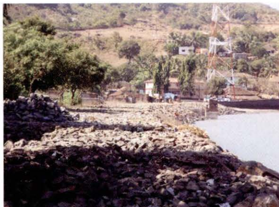
New approach road at Dighi – still in progress
