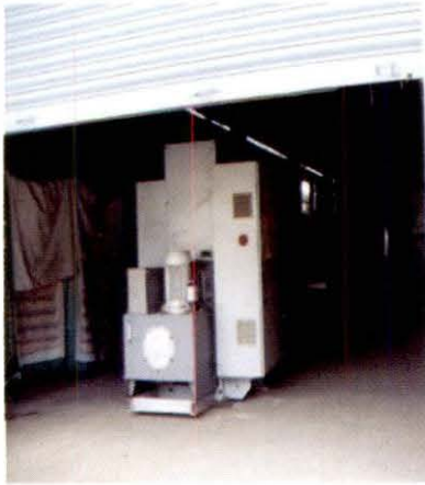
CTC machinery lying packed & unused at Auto Cluster, Vijaywada
