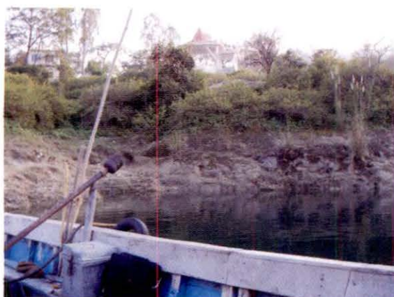
Terminal approach at Challelaghat not constructed
