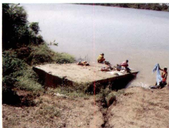
Jetty at Gangabet not in operation
