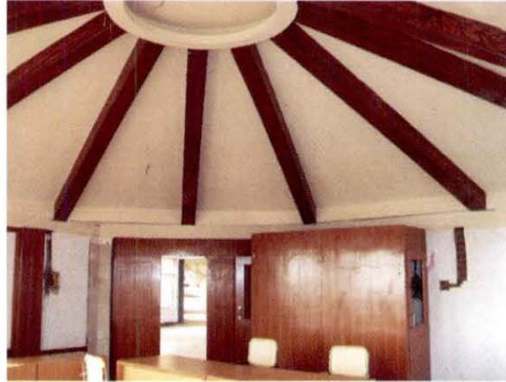
First Class and VIP Waiting Hall at Mandwa
