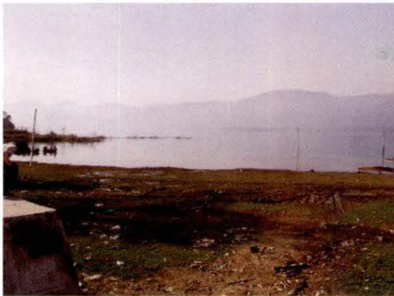
Jetty at Luhnu not constructed
