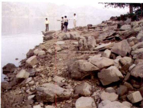
Small jetty at Nakranaghat not constructed
