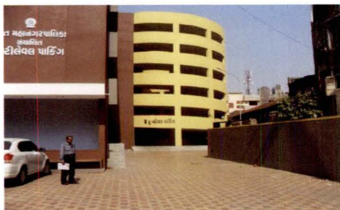
Multi-level parking being operated by SMC
