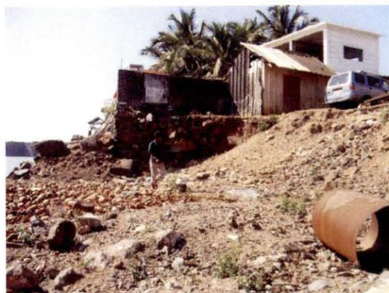
Existing Waiting Shed at Rajpuri dismantled
