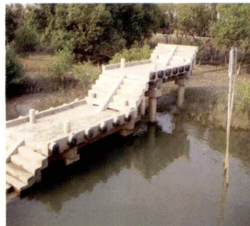
Jetty at Satjelia without approach road
