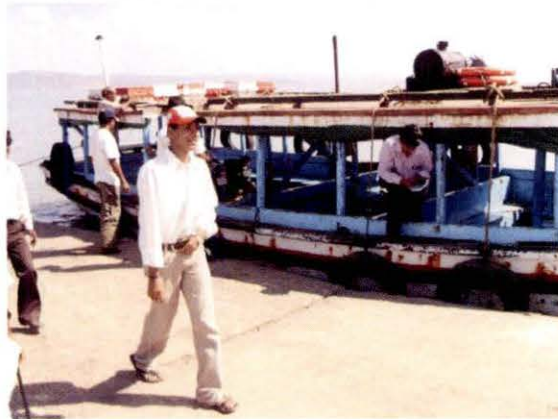
Existing jetty at Dighi
