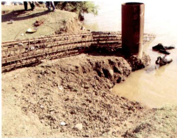
Proposed Jetty at Rahati – work started and stated to be nearing completion, but evidently not in progress
