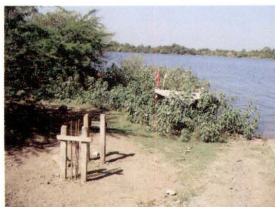
No approach road for jetty at Markand
