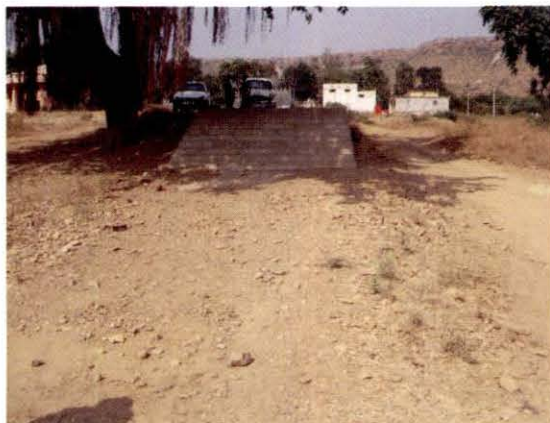
Rampura Jetty far way from water
