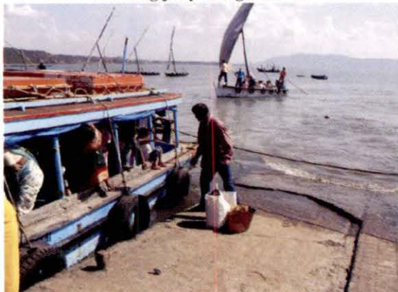
Existing jetty at Rajpuri
