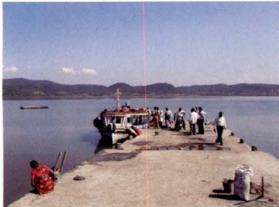
Existing jetty at Agardanda
