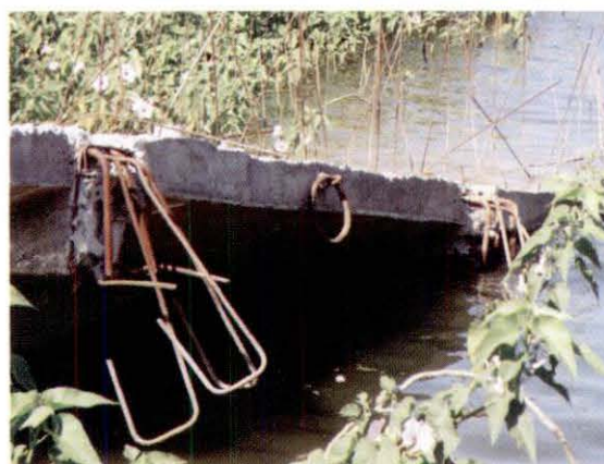
Jetty at Markand stated to be completed, but needing finishing, railing and steps
