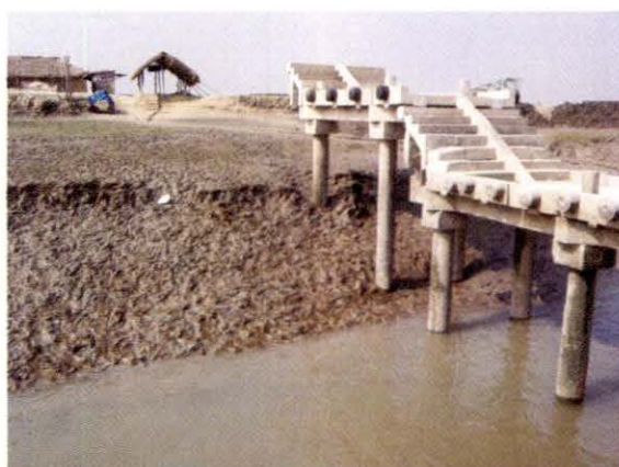
Jetty at Hogalduri without approach road
