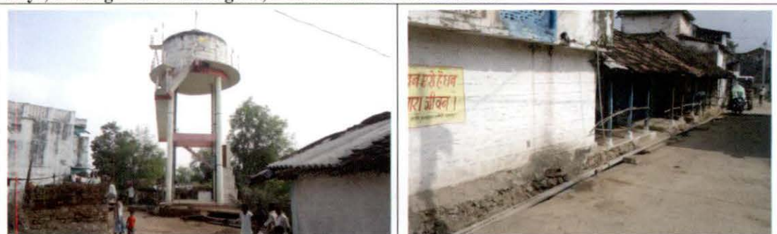
Over Head Tank constructed and GI pipeline can be seen layed at a cost of ₹ 6.50 lakh in October 2011 within village Ratanpur Girdhari, Raisen District from where household connection are provided. The PWSS is handed over to Mendki Panchayat of the village, having 115 individual household connections.
