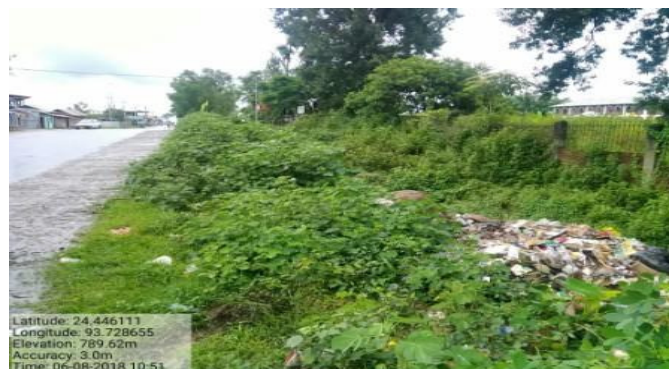
Dumping of waste on the roadside (Kwakta MC) (06 August 2018)
