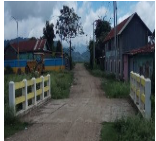
Bridge at Bisnunaha constructed with RIDF funding for bridge at Khoirom (20 August 2018)
