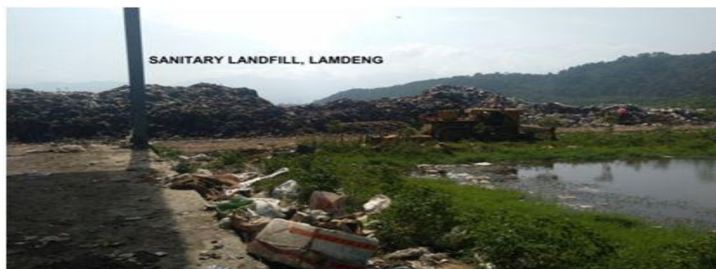
Uncompacted garbage dump height above 10 feet (20 June 2018)
