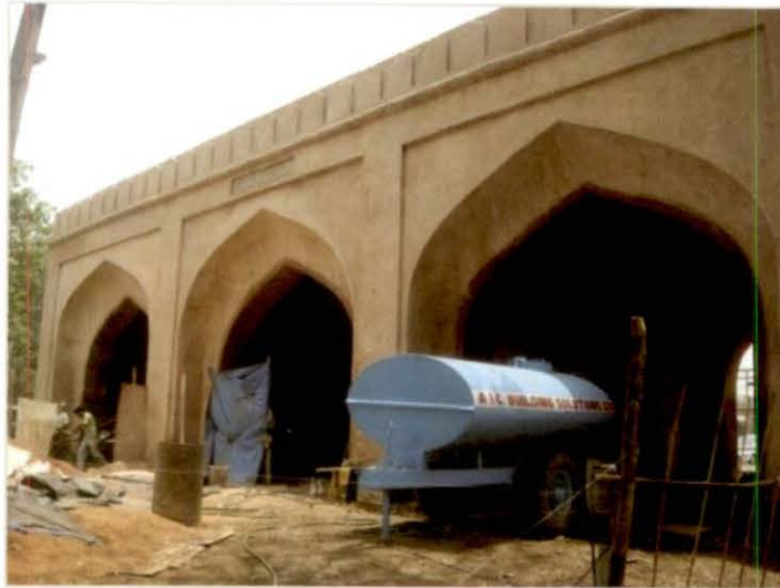
Tripolia Gate after conservation (missing designs)
