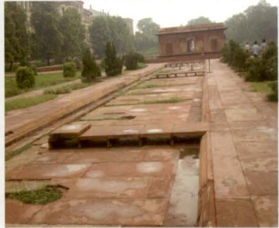
Improper maintenance of Hyat Baksh garden
