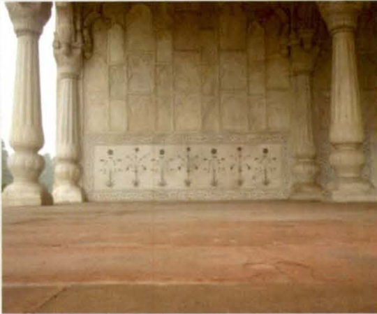
Inlay work carried out at Sawan Pavilion
