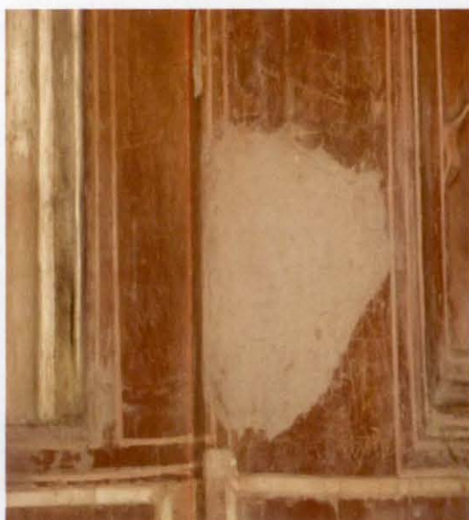
Cement work on wall in the mosque
