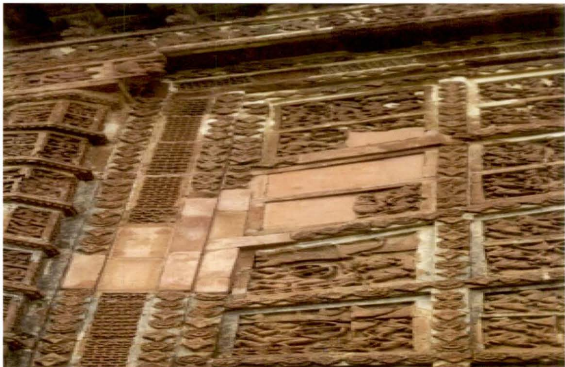
Patch work carried out at Jor Bunglow, Bishnupur, Kolkata Circle
