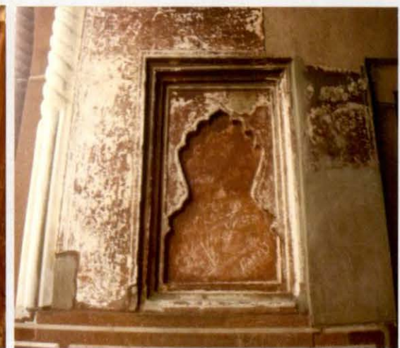
Fading of plaster of Paris in the Mehman Khana
