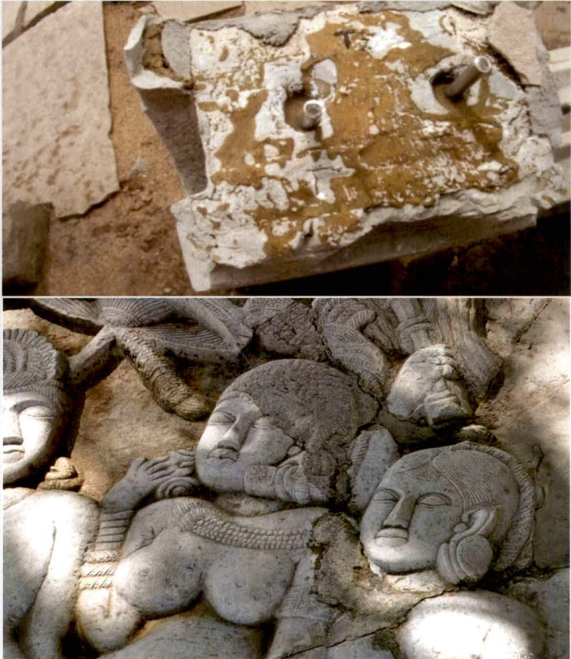
Faulty Repair works at the site
