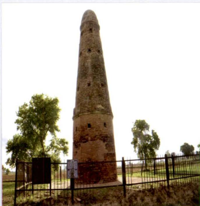
Dilapidated condition of Kos Minar No. 24, Banchari
