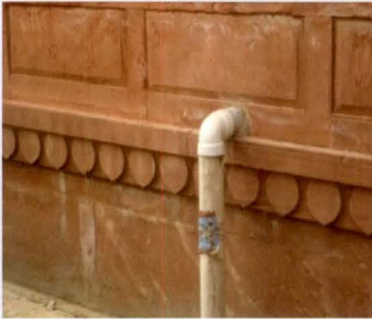
Plastic pipe fixed in the wall
