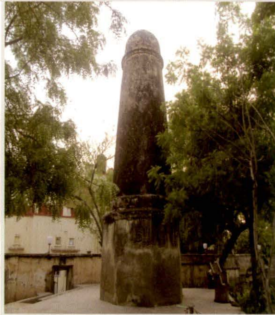
Kos Minar at Jaipur – Ajmer Road, Ajmer encroached by the residence of SP, Ajmer
