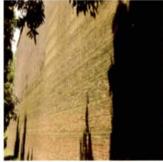
No recess in the reconstructed wall
