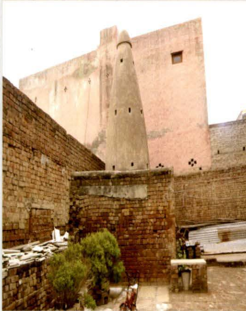
Kos Minar No. 26, Hodal encroached by a house
