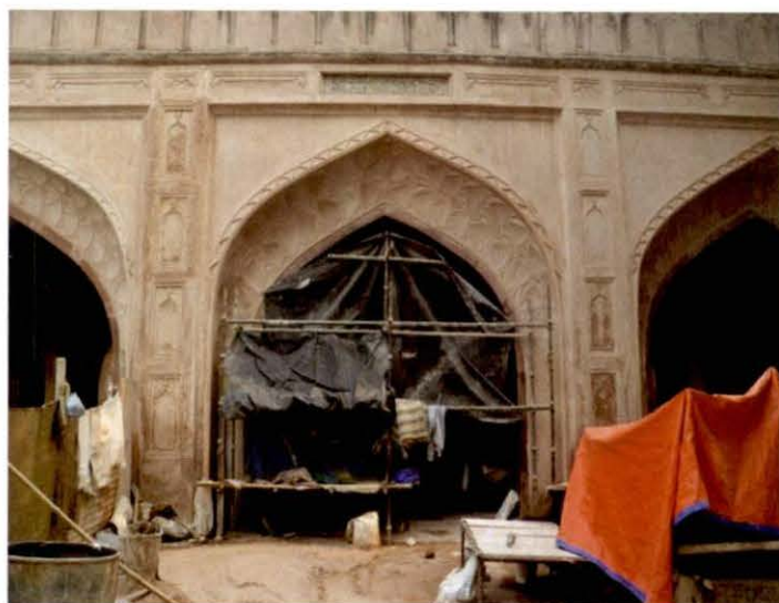
Tripolia Gate before conservation
