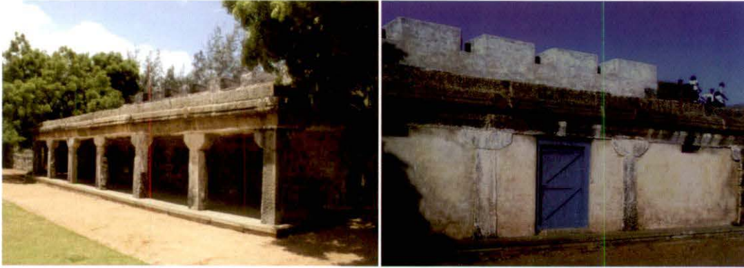
Mandapa's original look and after conversion to store house
