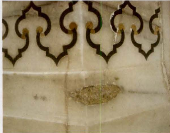
Patch work on the marble design
