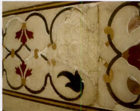
Patch work of the inlay work
