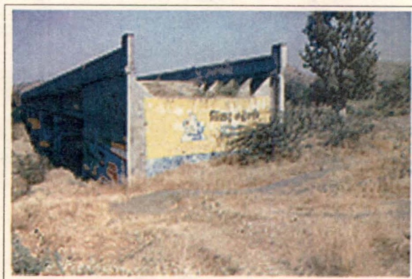
MESHWO BRIDGE MODASA APPROACH
