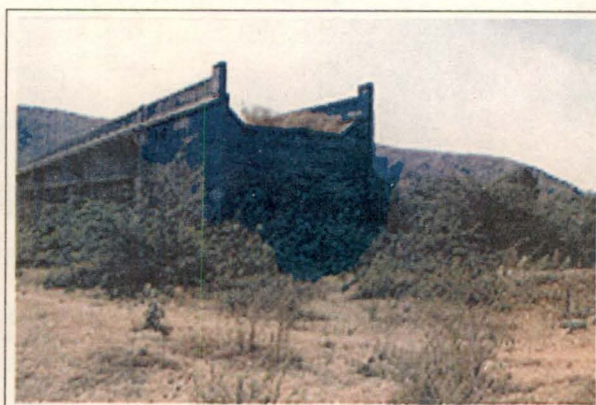
MESHWO BRIDGE SHAMLAJI APPROACH
