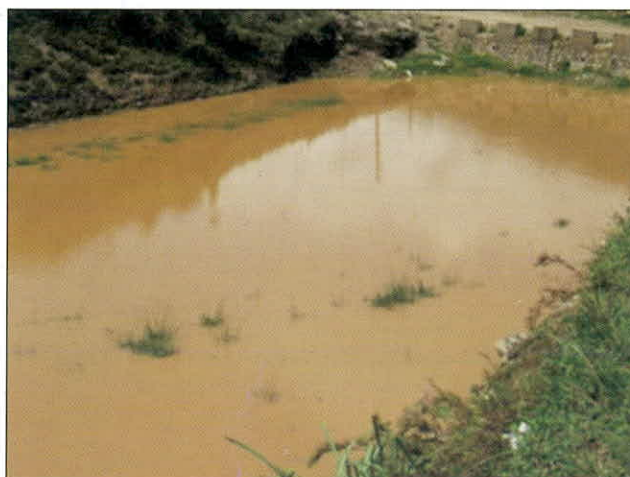
Waterlogged playground Pachey JHS, East
