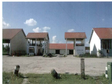
Checking Ramps for inspection of vehicles at Srirampur Composite check gate, Assam
