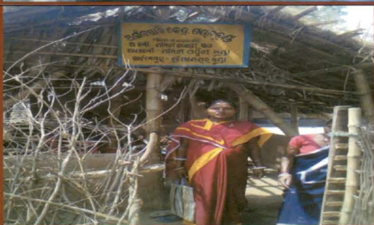
Exhibit 4.9 An Anganwadi Centre functioning in a thatched house exposed to sun, shower and cold in Keonjhar district, Odisha
