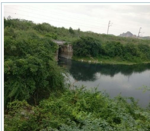
Effluents of dyeing units flowing through municipal drains into Nagari tank
