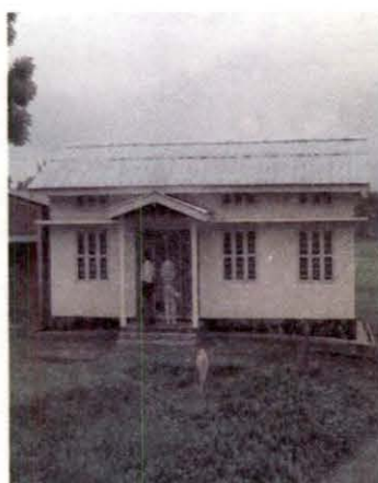
Newly constructed Khanajan Sub Centre in Assam
