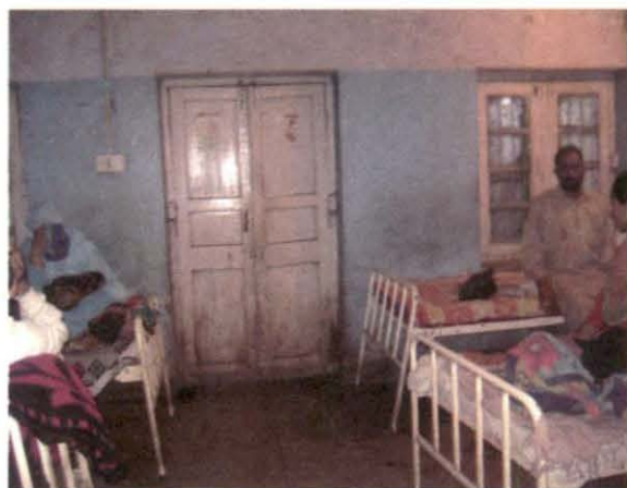
Poor condition of maternity ward at District Hospital, Rajouri, Jammu and Kashmir
