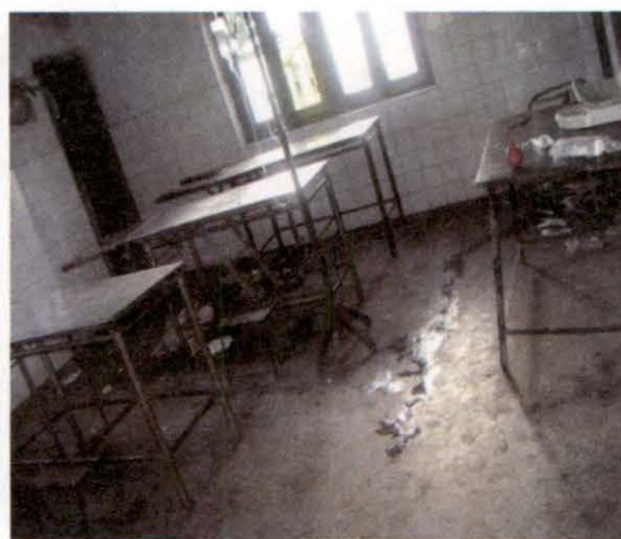
Unequipped Operation Theatre of PHC Piro, Bihar
