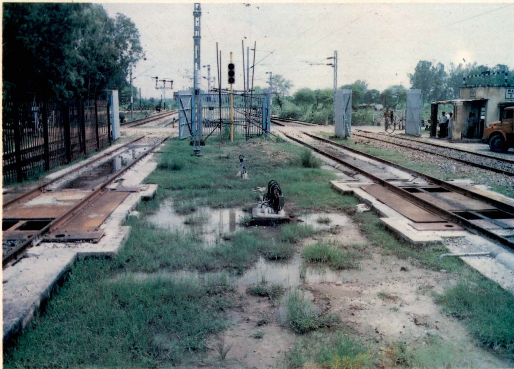
A view of two Electronic in-motion weigh bridges installed on reception lines for weightment of full rake of coal wagons.
