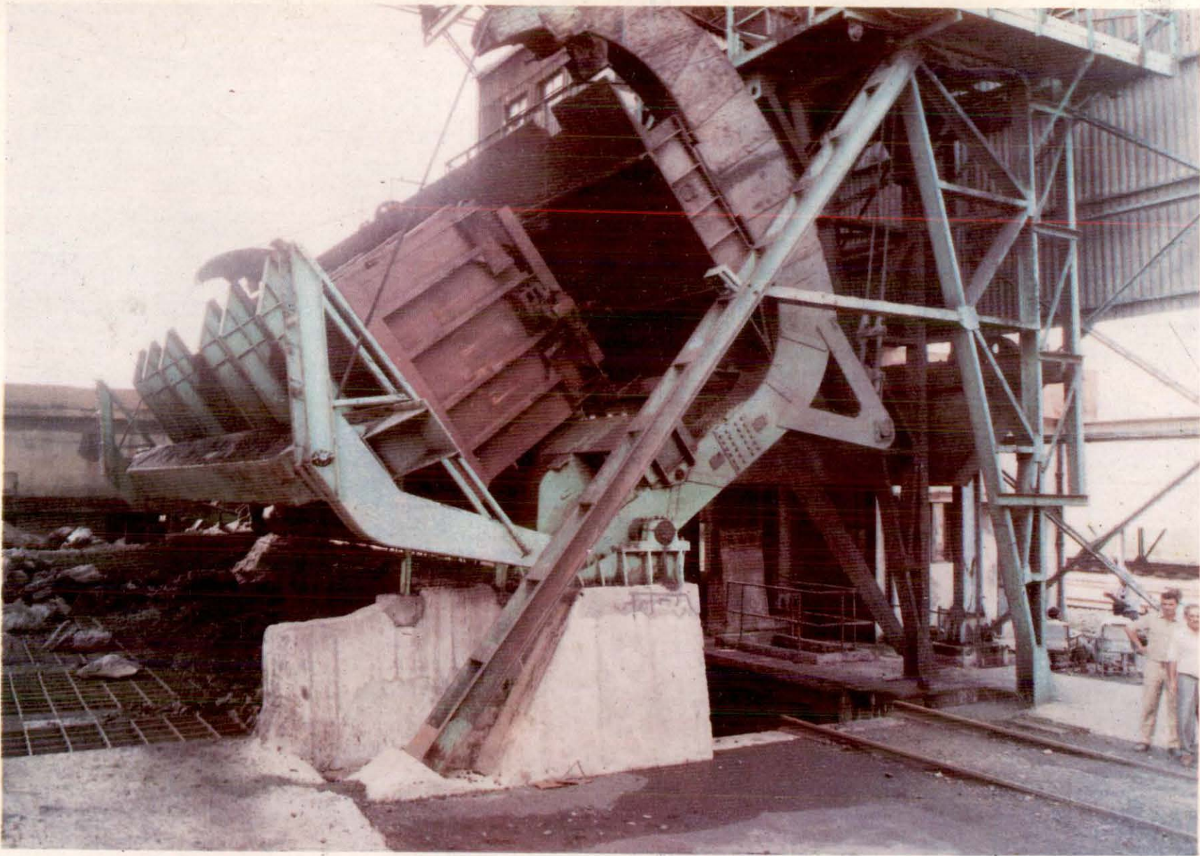
A view of wagon tipplers for unloading coal on common hopper from conventional railway wagons.
