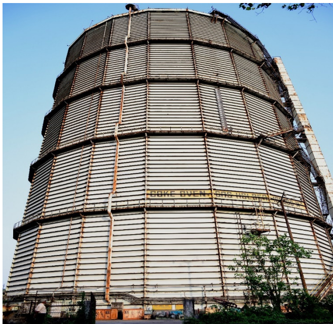
Figure 5.1: Coke Oven Gas Holder
