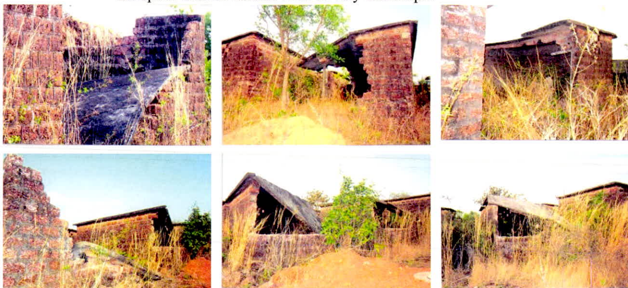
(Collapsed roofs and walls of Ashraya houses)
