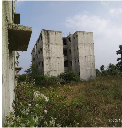
Partial super structure 1BHK block
