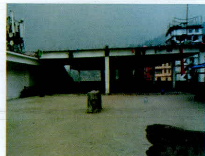
Idle and incomplete structure for Call Centre
