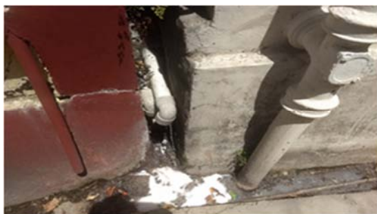
Grey water pipe being discharged from households into the storm water-drains in Sundernagar (14.05.2018)
