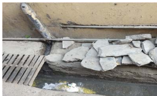
Grey water pipe being discharged from a household into storm-water drains in Chamba (06.04.2018)
