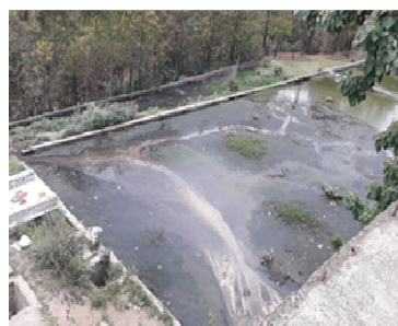
Uncovered sludge drying beds inundated/ overflowing with water at STP, Shamti, Solan (05 June 2018)
