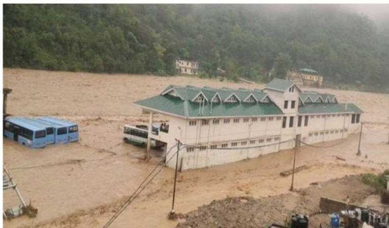
Photograph showing damage caused to Dharampur bus stand and buses due to flash flood during intervening night of 7-8 August 2015 as a result of construction of bus stand amidst the khad without flood protection measures.
