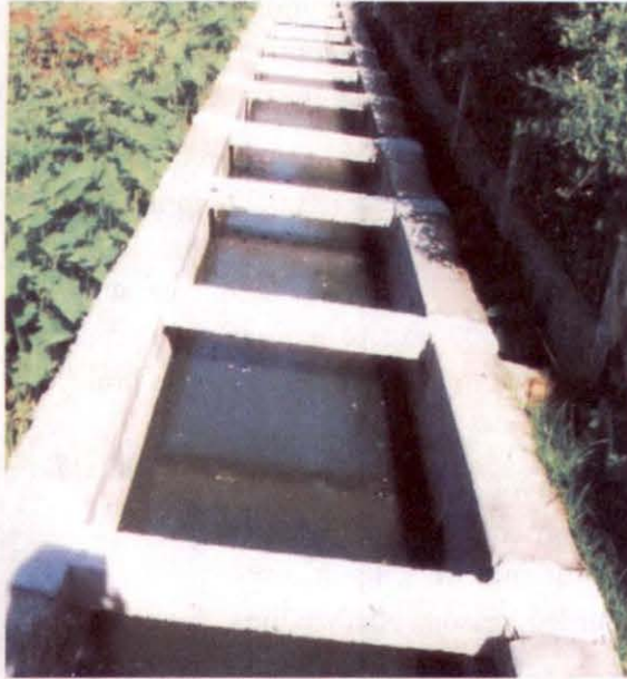
Drain No-7/Along Chandmari Bye Lane No-2
