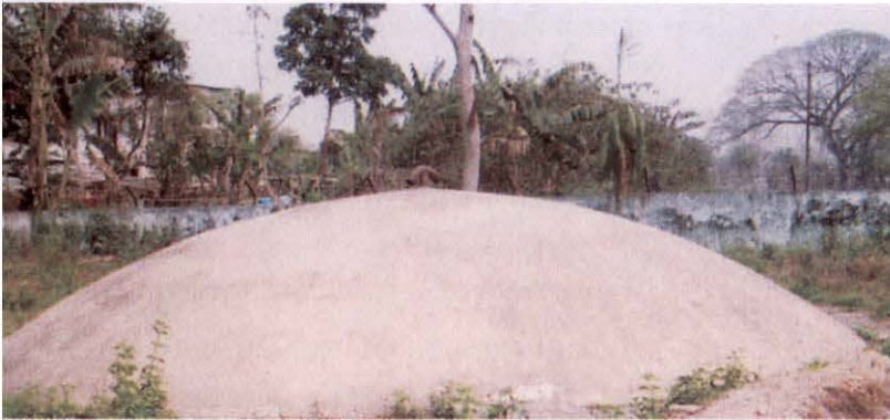
Clear water sump of Dergaon TWSS
