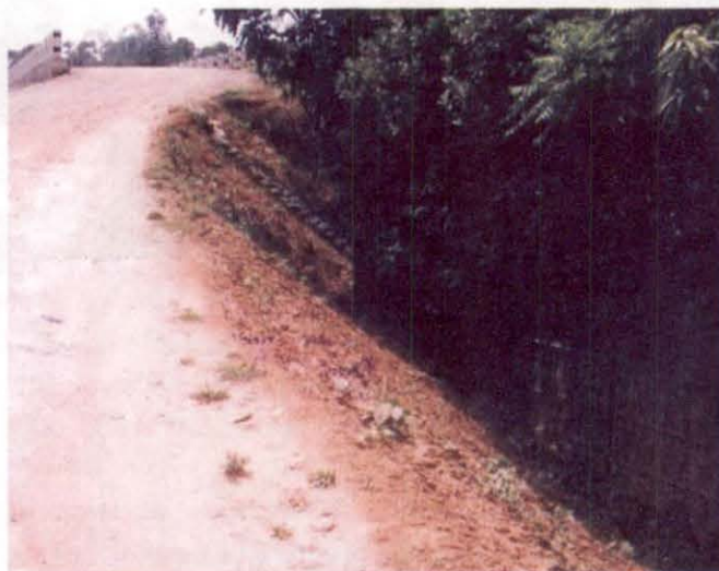
RCC Bridge No. 15/1 on Silchar-Kumbhirgram Road
