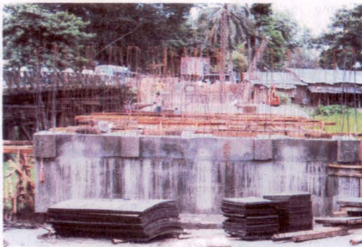
RCC bridge No-1/1 over river Shantijan
