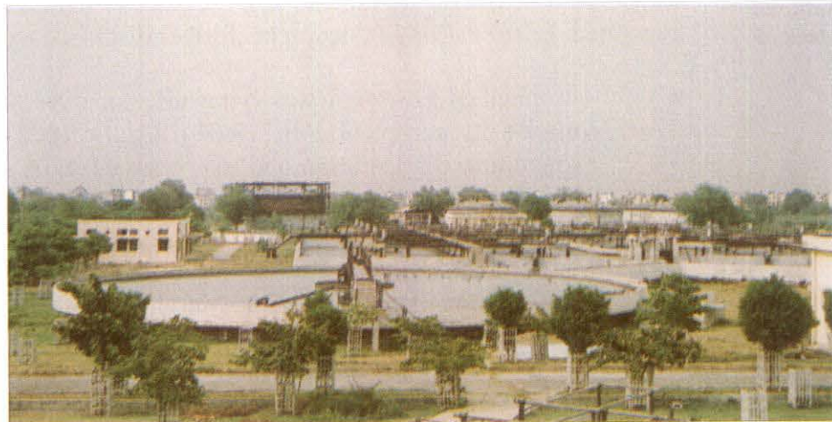
Figure-6: A view of Okhla STP
