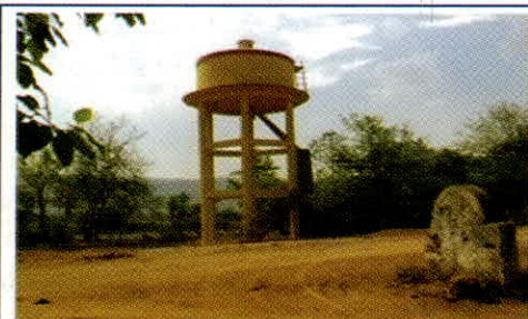
Elevated storage reservoir of RPWS to Makarsala in Kalahandi district without pump house and external electrification works
