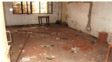
Condition of rooms
