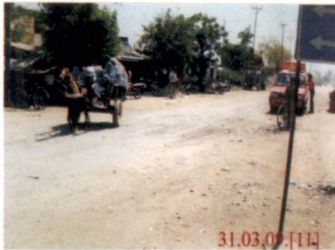
Bajpur-Janginala road – At Km 3
