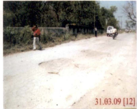
Bajpur-Janginala road – At Km 4
