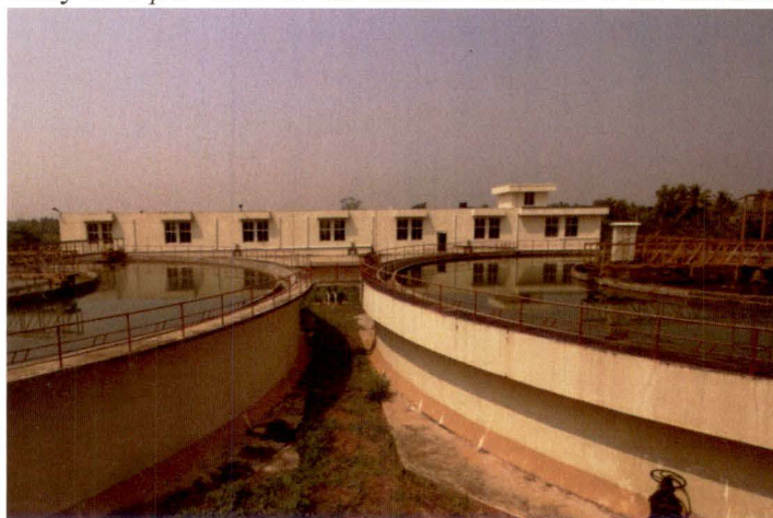
Completed water treatment plant remaining unutilised
