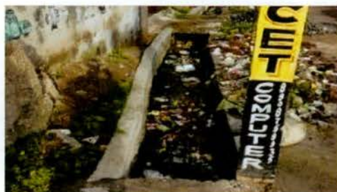
View of a choked drain
