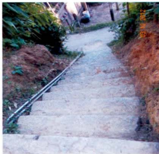
A photograph showing Construction of Stone Masonry steps with chequered tiles from Mawitea's house to K. Lalrinzuali's house, Luangmual (no chequered tiles provided)
