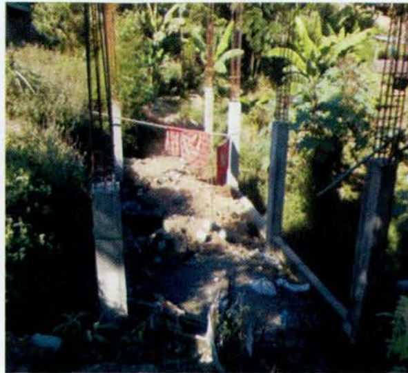
A photograph showing incomplete status of Construction of Community Hall, Phungchawng.
