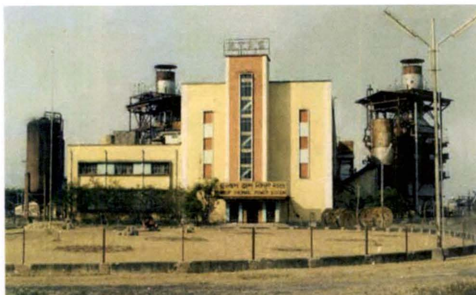
NAMRUP THERMAL POWER STATION
