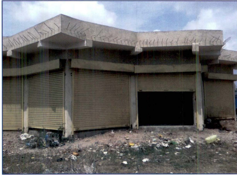
Picture 4: Renovated Zadeshwar village haat (02.07.2014)
