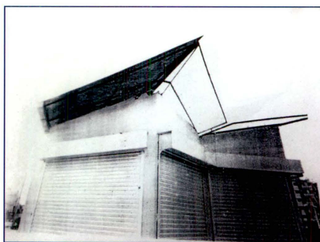
Picture 3: FRP sheet damaged/blown during monsoon at Zadeshwar village haat (Picture taken from file)
