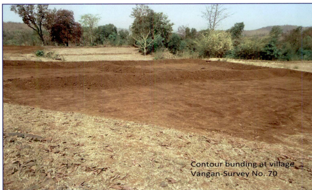
Picture 13: Contour bund constructed under IWMP-1, Navsari district (from the records of DWDU)
