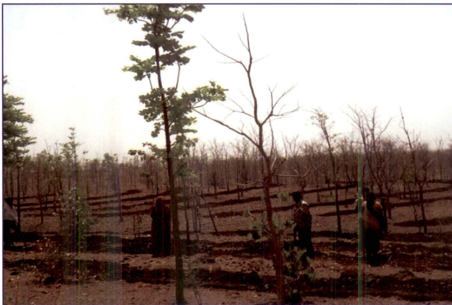
Picture 5 : Contour trench constructed in area without adequate slope in IWMP-3 of Dahod district (03.09.2014)
