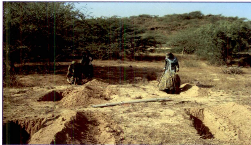
Picture 3 : Contour trench constructed at foothill and parallel to water flow instead of perpendicular to water flow in IWMP-1 of Kachchh (photo taken at the time of completion of construction work obtained from the records of DWDU)
