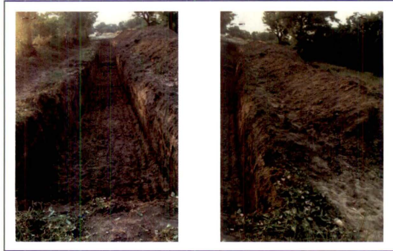
Picture 2 : Staggered Contour trench at village Bhojva in IWMP-8 of Ahmedabad (photo taken at the time of completion of construction work obtained from the records of DWDU)
