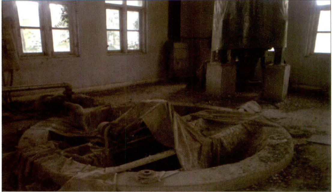
Non-operational Paper Pulp Plant
