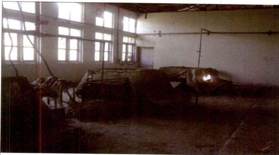
Non-operational Carpet Washing and Drying Plant
