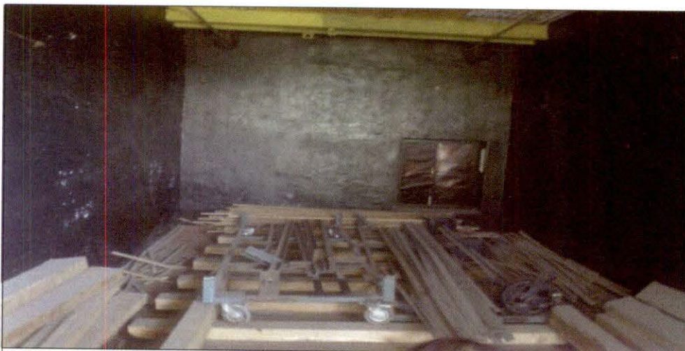
Non-operational Wood Seasoning Plant
