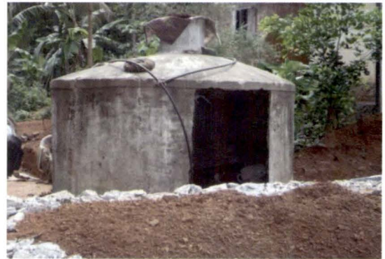
Figure 3.1: Abandoned Rain Water Harvesting Structure, Peruvampadam ST Colony
