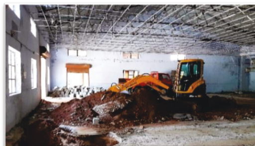
Fig: 4.2 Civil work at CSP Kuttur
