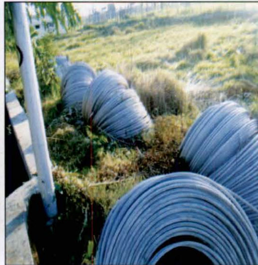
ACSR conductor lying in open place at 400 KV SS, Kashipur
