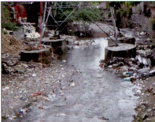
File photo of position of tower with foundation at Bindal River, Dehradun
