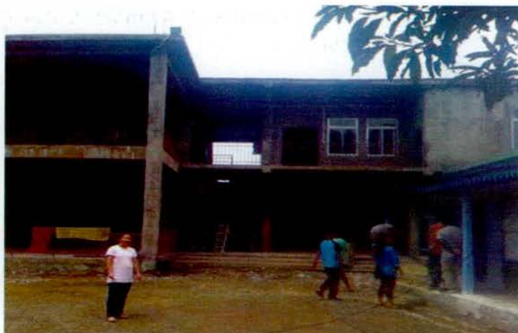
SDH Khawzawl under construction
