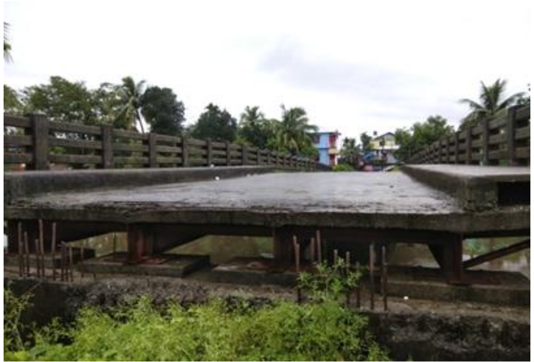
Pic 3.1: West side of the bridge
