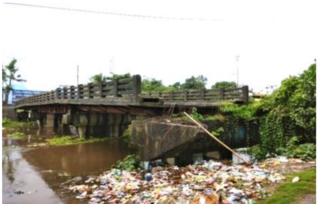
Pic 3.2: East side of the bridge
