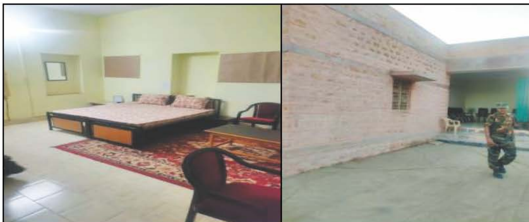
Construction of two mini wards, one cool room, staff office and Medical Officer's room with toilets Ghotaru, GP Shahgarh, PS Sam, ZP Jaisalmer (Work ID:2017-18/13281) (Completed: November 2018). Date of Physical verification-23.09.2021
