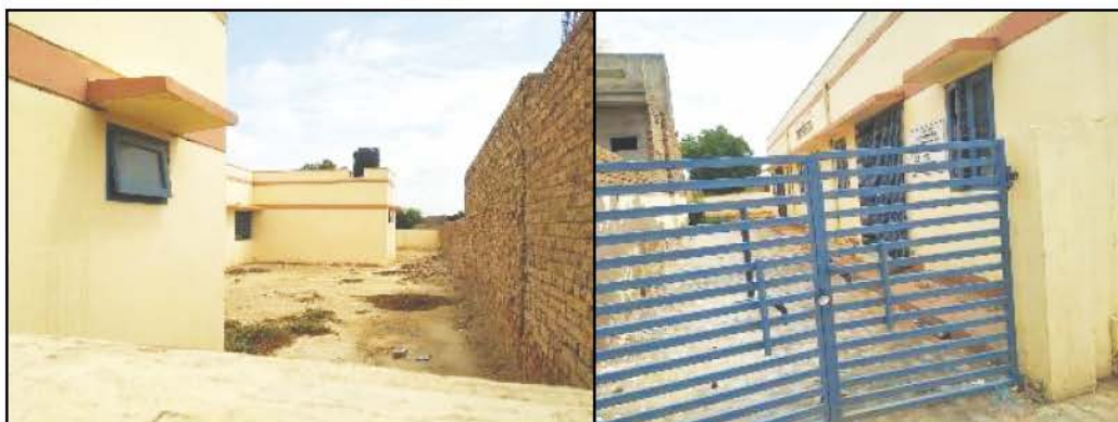
Construction of 10 bedded AC Hospital in village 27-A near BOP Kailash, GP 27-A, PS Anupgarh, ZP Sri Ganganagar (Work ID:2019-20/333) (Completed: March 2021). Date of Physical verification- 23.09.2021.
