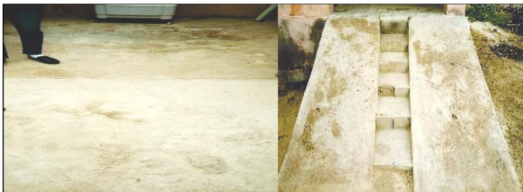
Construction of teacher's house in Government Upper Primary School, 12 KYD, GP: 17 KYD, PS: Khajuwala, ZP: Bikaner (Work ID: 2016-17/19995) (Completed: July 2018). Physical Verification during 31.08.2021 to 06.09.2021.
