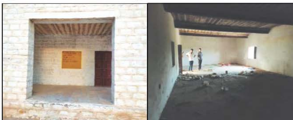
Construction of Computer Room at Government Senior Secondary School, Raymala, GP Raimala, PS Sam, ZP Jaisalmer, (Work ID: 2017-18/18779) (Completed: September 2018) Date of Physical Verification 14.09.2021
