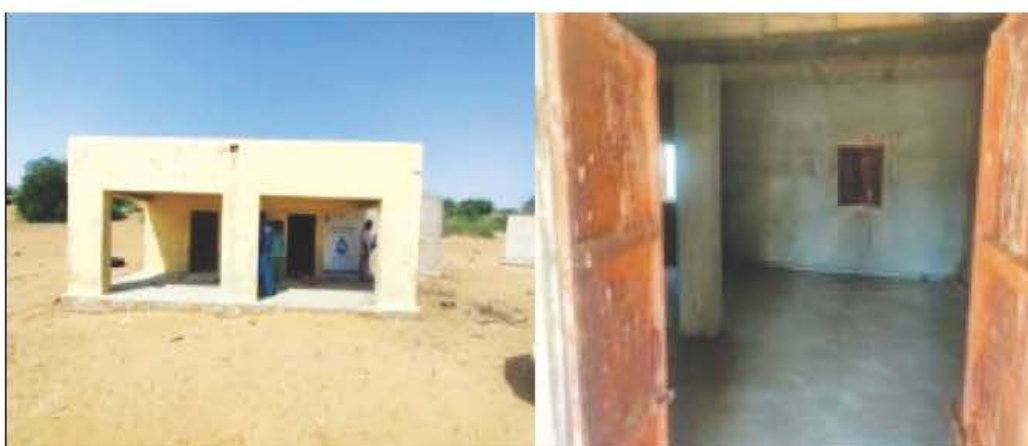
Construction of additional classroom, Government Primary School, Murar, GP Harnau, PS Sam, ZP Jaisalmer (Work ID: 2018-19/29557) (Completed: September 2019). Date of Physical Verification 05.10.2021.
