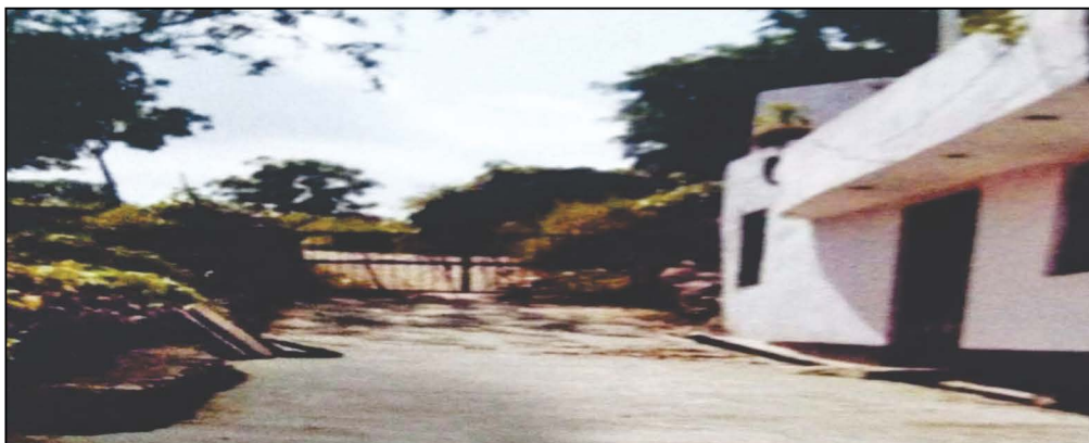
Case 4: Encroachment (October 2019) on the road by fixing an iron gate in the middle of the road.
