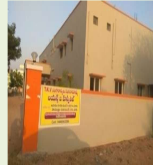
Figure-3.8: Construction of OP block in private land (02 May 2018)
