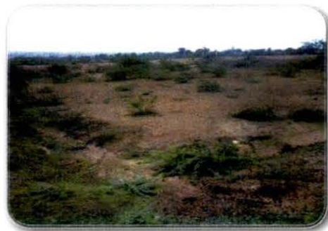
Picture 19 Incomplete SLF developed by GUDC, under GERRP at Bhachau, Kutch District (10.07.2013)
