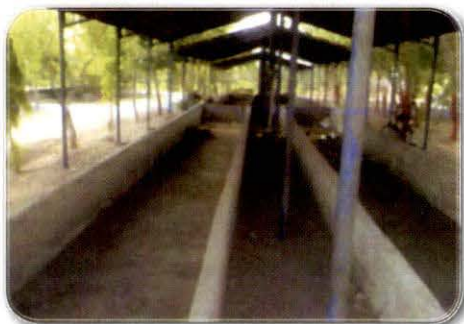
Picture 12 VCP at Bagsara NP, Amreli District (05.06.2013)
