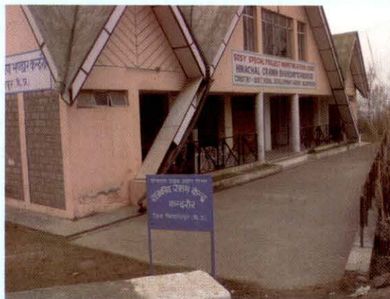
Portion of GHB at Kandraur rented out to General Manager, District Industries Centre
