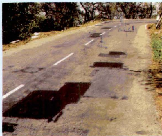
Mubarikpur-Ranital-Kangra road (km 117/635)
