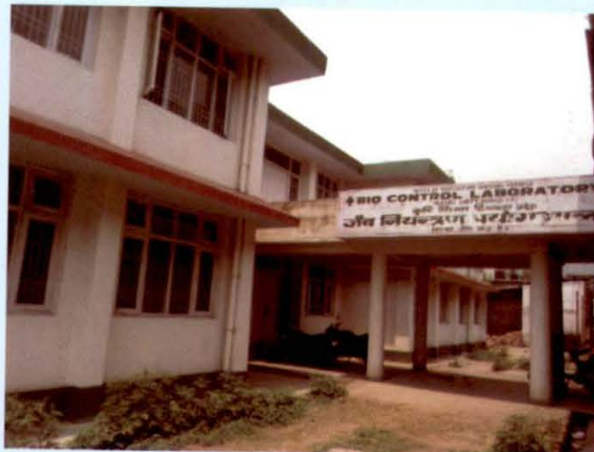
Building constructed for setting up of State Bio Control Laboratory at Mandi
