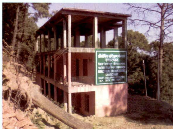
Partially completed GHB at Swarghat, Bilaspur District
