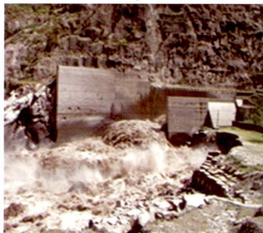
Flood water discharge form Radial Gate
